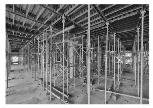
Green formwork system usage is similar to aluminium formwork and are primarily used for building / formation of horizontal structures (e.g. floors). It is a panel-drop concrete formwork system with early-stripping mechanism. It provides a systematic, modular formwork solution for the construction of beam and slab structural elements and suits generally all in-situ construction methods and conditions.
