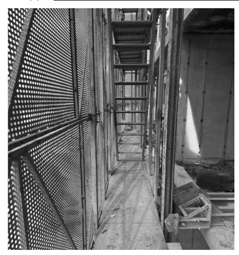
The scaffolding is a self-climbing protecting screen with working platform and comes equipped with controlled, synchronised climbing mechanism designed to prevent workers and objects from falling when working at heights.
